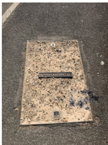
Image 2). Pavement not suitable for wheelchair user as raised manhole cover
